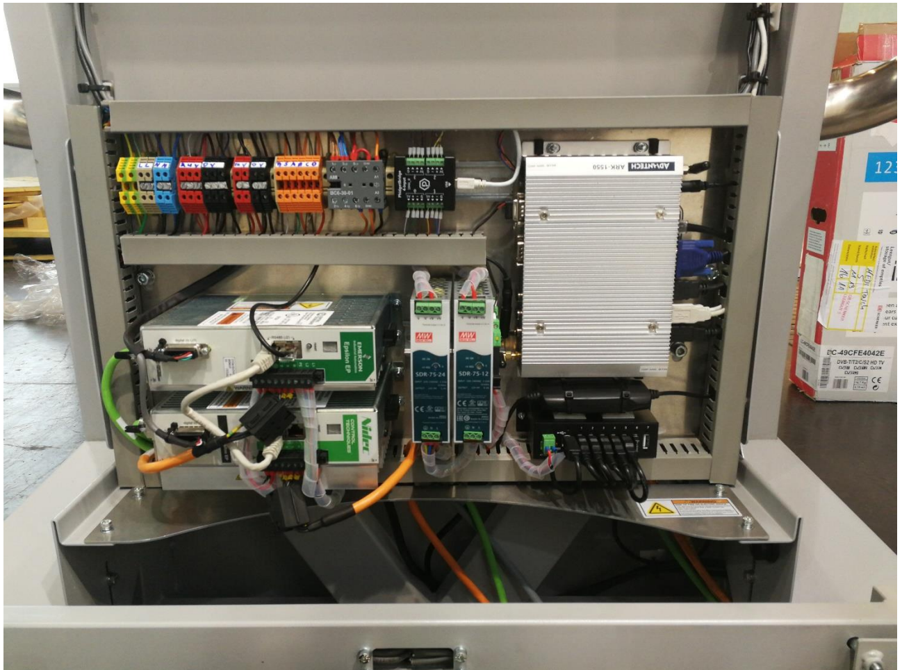
Fig.3 General internal view
